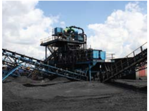
Black Wattle Dump, a reclamation operation managed by Zingaro Coal reclaims coal from the Black Wattle Colliery in Witbank, Mpumalanga
